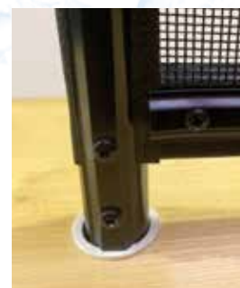
Drilling \varnothing 30 mm
